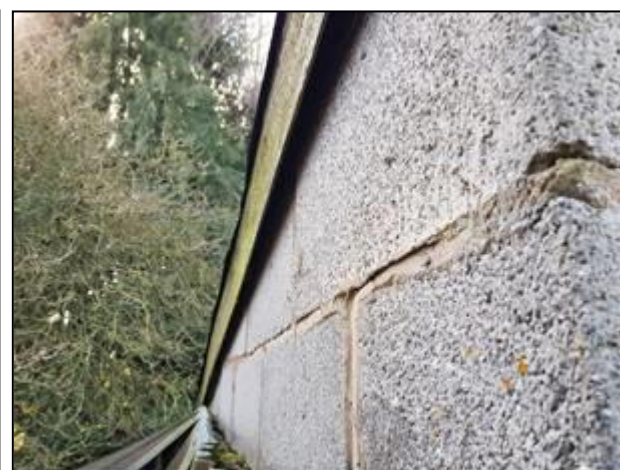
Photo 9 – Gaps unsuitable / debris-filled at verges
